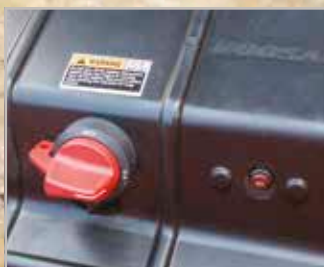
Battery cut-off switch
